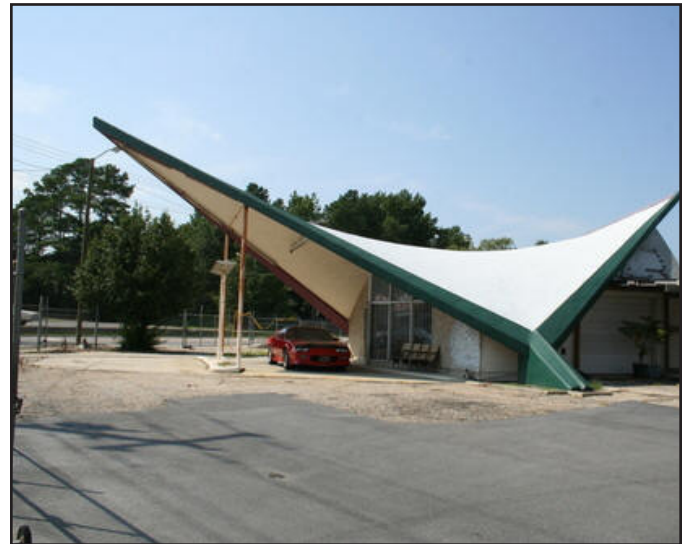
Fig. 9: Pam-Oil Gas Station, Fayetteville, NC
