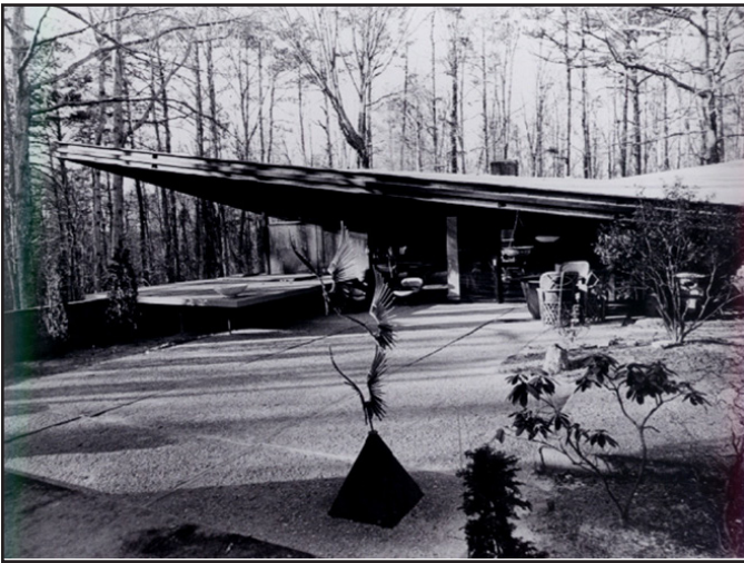
Fig. 4: Patio of Catalano House, Raleigh, NC
