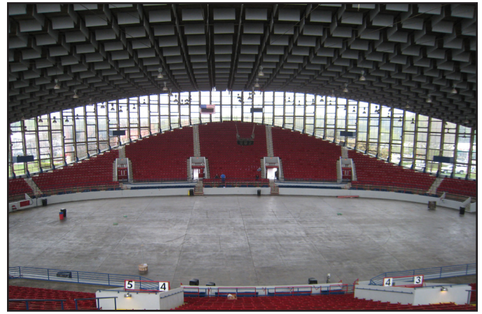
Fig. 7: Interior of Dorton Arena, Raleigh, NC
