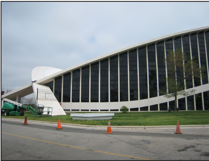
Fig. 8: Side of Dorton Arena, Raleigh, NC
