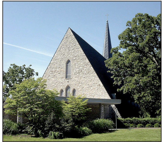
Fig. 9: Grace Episcopal Church in Kirkwood, Missouri is an example of a suburban A-frame place of worship.
