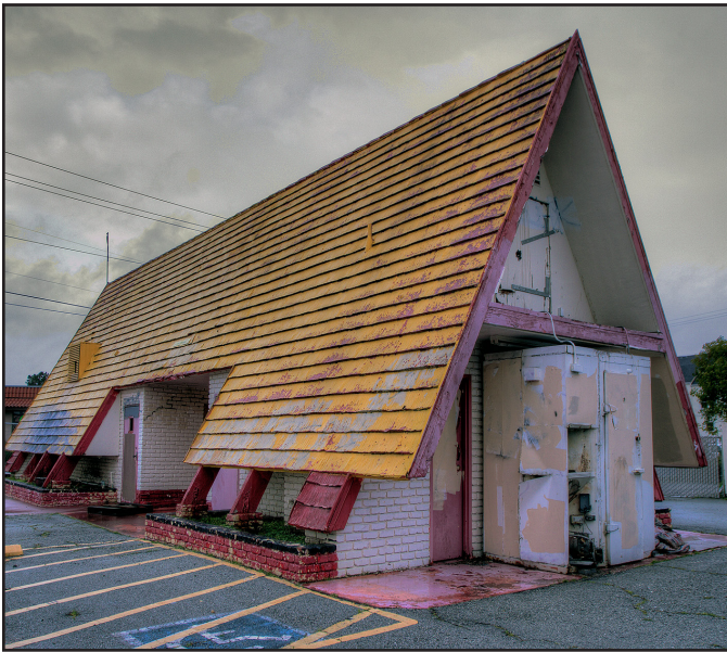
Fig. 8: The California chain Der Wienerschnitzel utilized a false A-frame structure with a center drive-thru.
