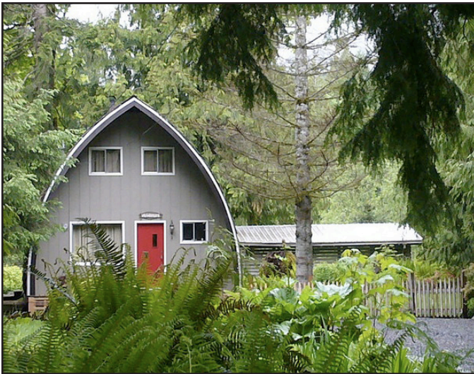
Fig. 2: The Arched or Gothic A-frame is one variation that seeks to create a more spacious second floor.
