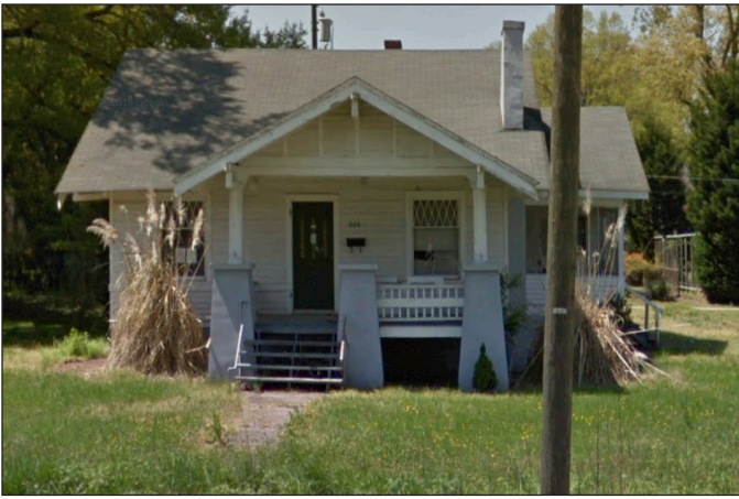
Fig. 18: The Pomona model at 909 Madison St., Roanoke Rapids has an addition on the right elevation.
