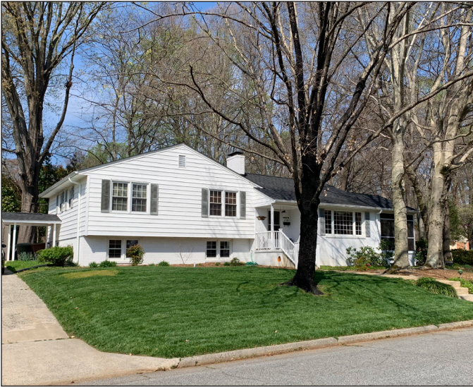
Fig. 10: Split-level house with exterior updates
