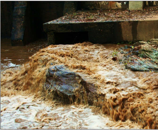
Fig. 10: Milldam gates open releasing a torrent of water and sediment from behind the impoundment.
