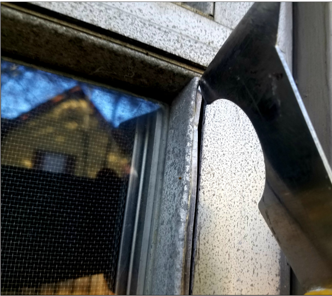
Fig. 8: careful removal of snap aluminum window glazing
