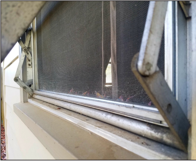
Fig. 10: Tru-seal torque bar and torque bar arm
