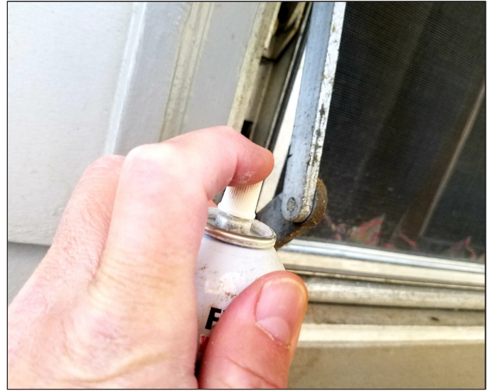
Fig. 11: lubrication of moving parts using dry lube
