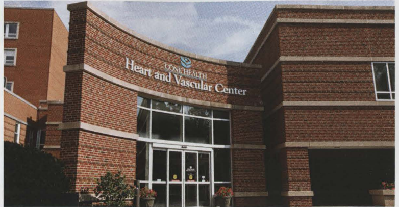
The Heart Failure Clinic is located in the Heart and Vascular center on the Moses H. Cone Memorial Hospital campus.
