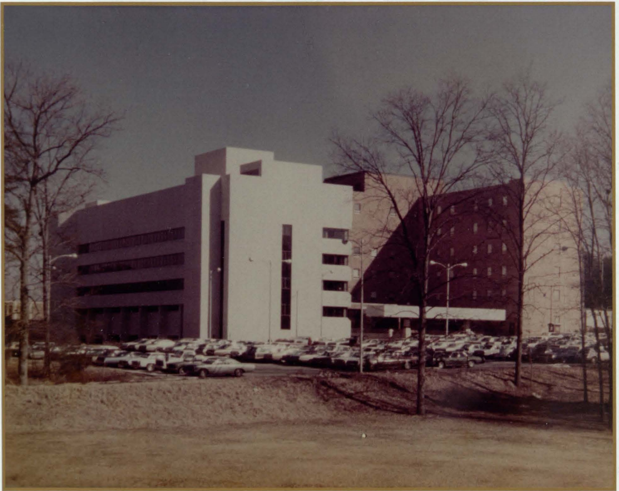
West Wing addition, 1976
