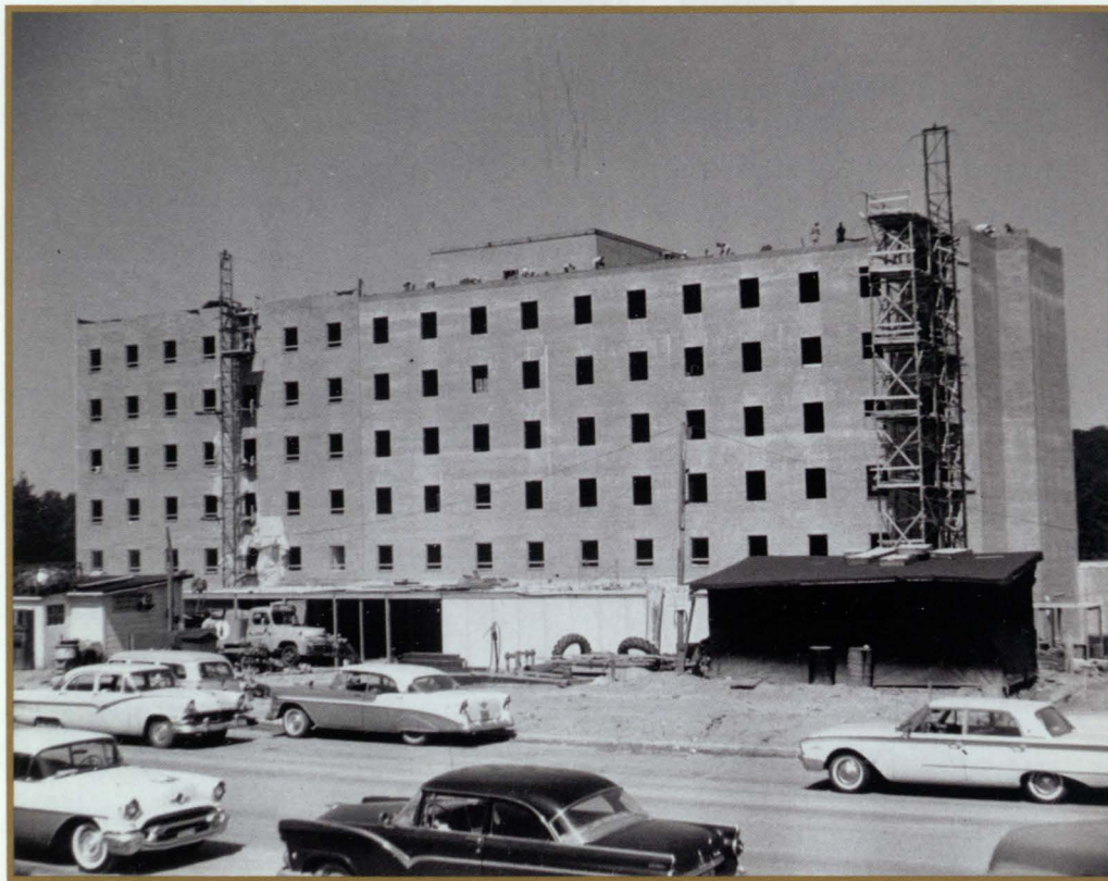
501 N. Elam Ave. building under construction, 1960
