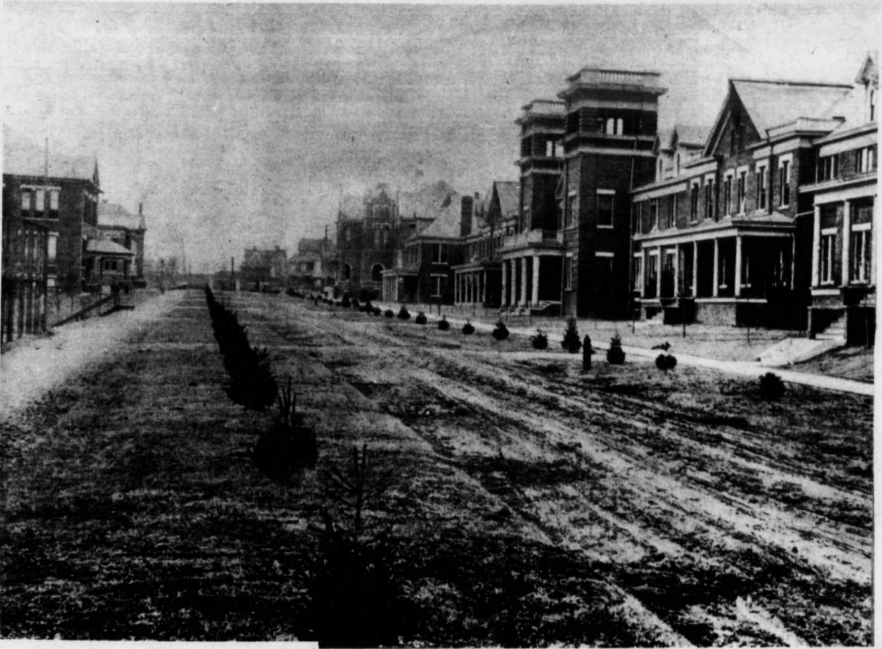
UNC - G'S FACADE HAS CHANGED GREATLY THROUGH THE YEARS AS SEEN IN THESE OLD PHOTOGRAPHS OF COLLEGE AVENUE (ABOVE)
