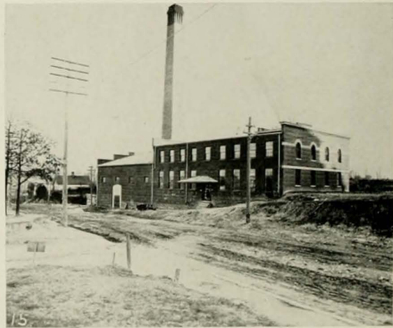
VIEW OF WALKER AVENUE AND THE LAUNDRY, 1904
