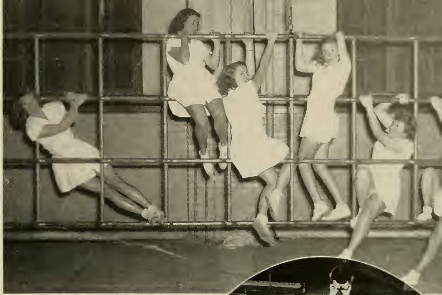
Work on the window lattice.
