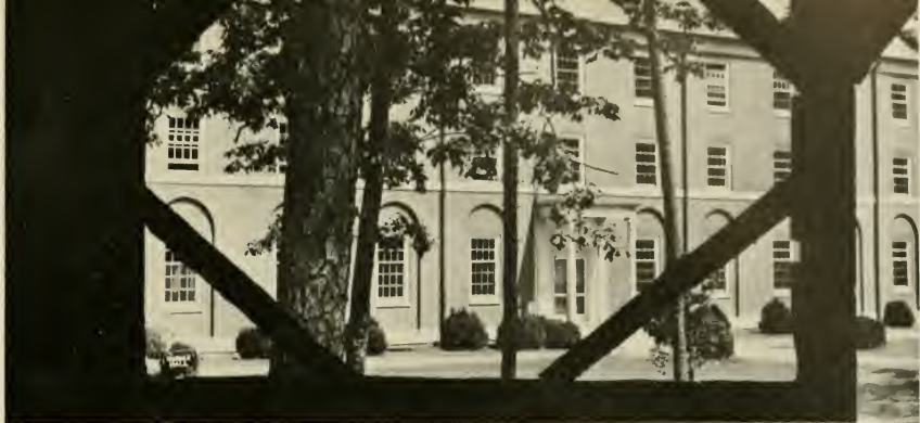
... And a sink in every room?
