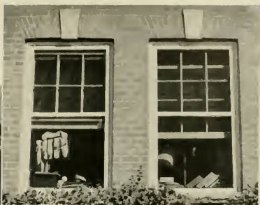
W.C. as viewed from the tennis courts.
