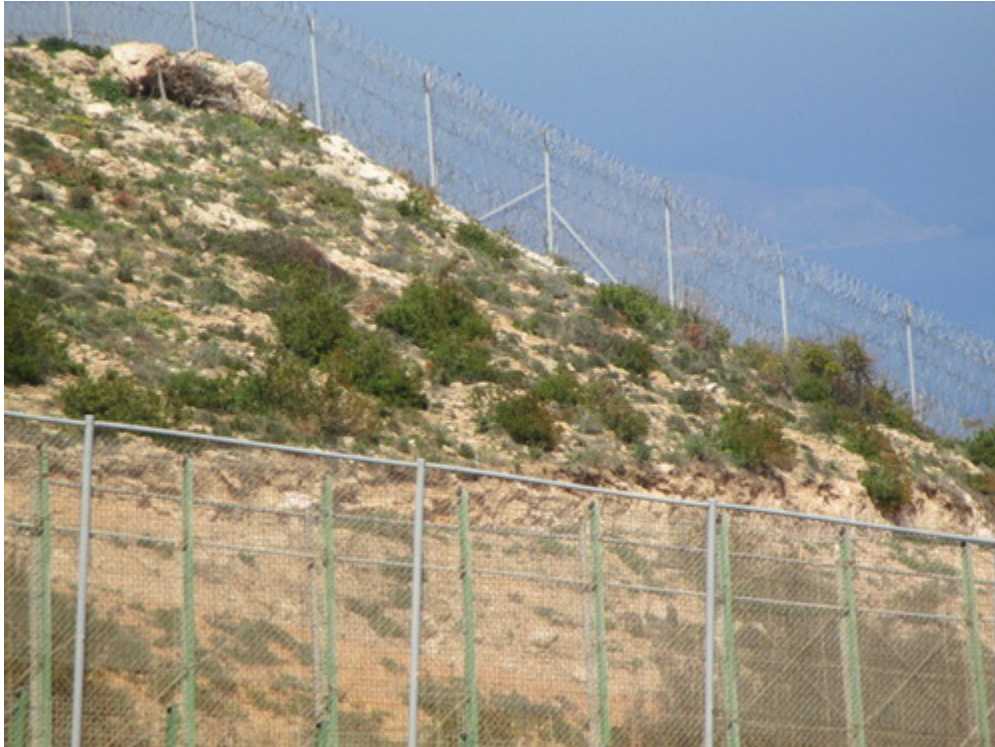
Figure 5. Spanish fences in foreground, new Moroccan concertina wire fence in background.
